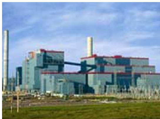
Genesee Thermal Generation Facility
