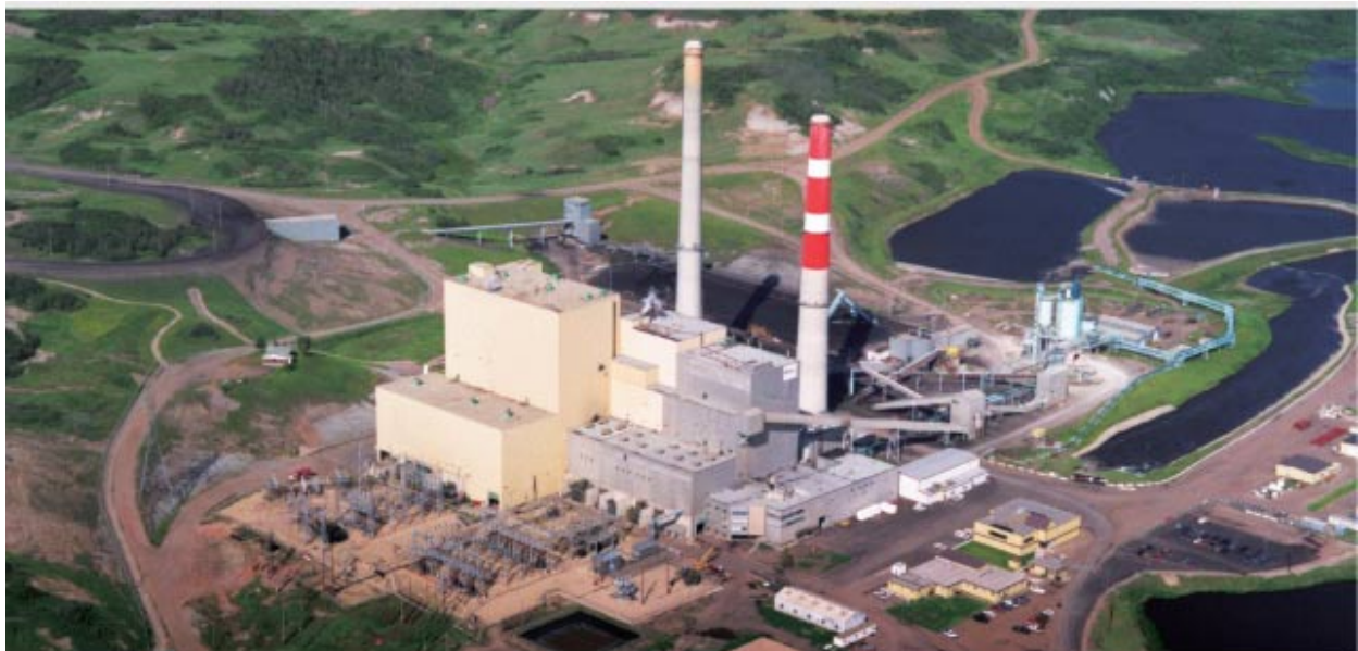
Battle River Thermal Generating Facility
