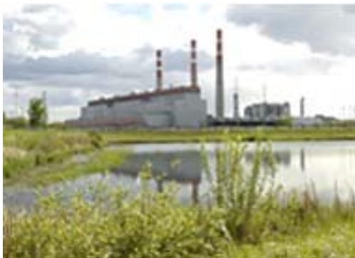
Sundance Thermal Generation Facility
