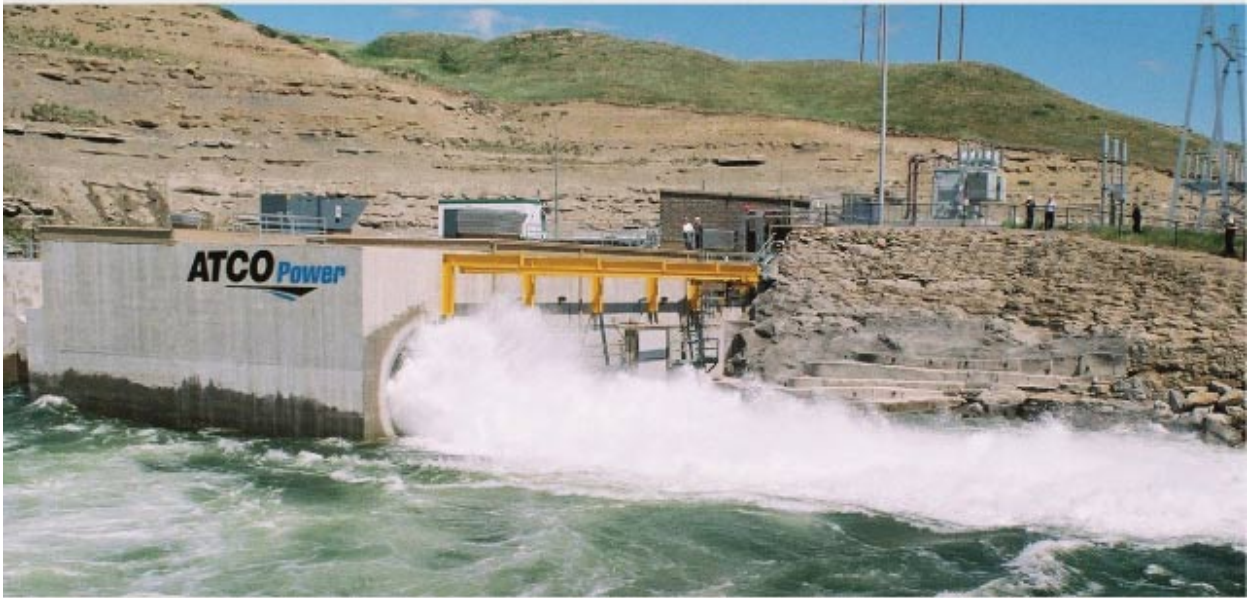
Oldman River Hydro Facility
