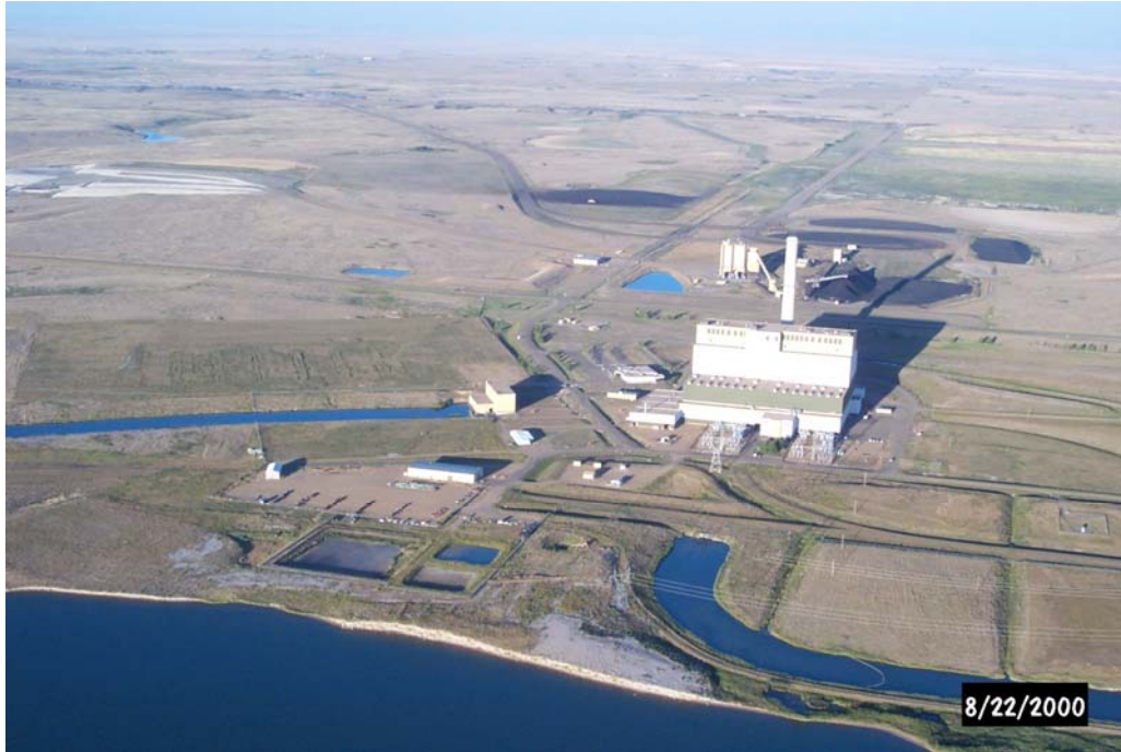
Sheerness Thermal Generating Facility
